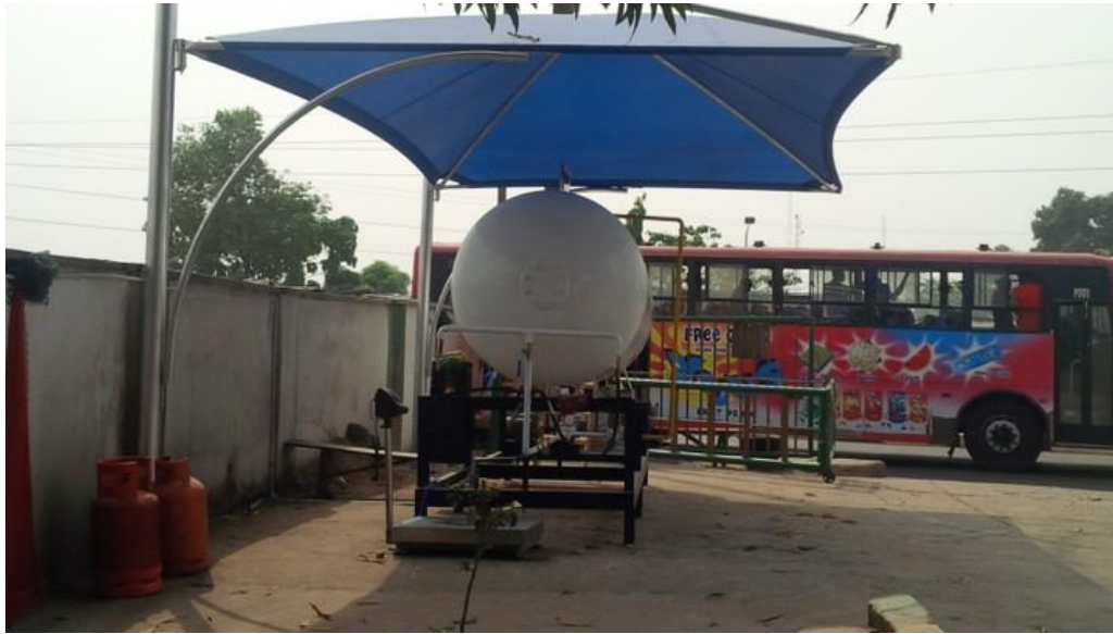
Fig 2. Sample of Storage for small scale as seen in Fuel stations. This has the facility to dispense direct to bottles and cost of setting this is =N= 15,000,000 . Including little land space.
